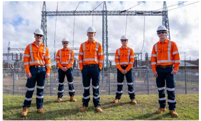
Five new Genus apprentices have begun work on the construction of the Hunter Coast Renewable Energy Zone network infrastructure project
