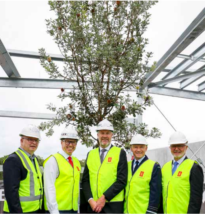
A ‘topping out’ ceremony was held onsite on 19 May, marking a major construction milestone for this complex manufacturing and maintenance facility.
